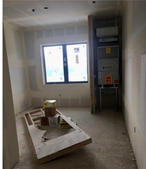
This month there has been a lot of progress on the third floor, which includes the sleeping rooms (pictured) in the domestic violence shelter wing. Individual heating and cooling units have been installed, so that each family will be able to control the temperature in their room. Drywall has also been installed. It's exciting to see the building's interior take shape!
